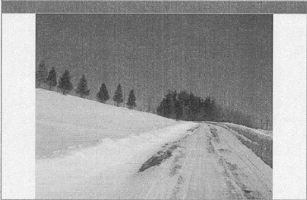
Bogner Drive Looking North (Site on Right)
